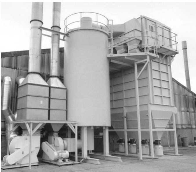
Figure 2.40 Carbon abatement unit for emissions from flexible polyurethane foam processing. Reproduced by kind permission of Camfil, Blackburn, UK
