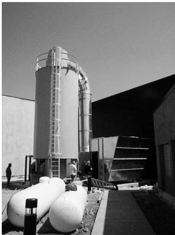
Figure 2.41 Carbon abatement unit for emissions from a polyurethane flame lamination process. Reproduced by kind permission of Camfil, Blackburn, UK
